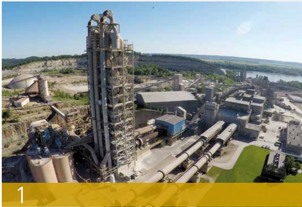
1. VISTA DELLA LINEA FORNO RIVER 7000 / VIEW OF THE RIVER 7000 KILN LINE
